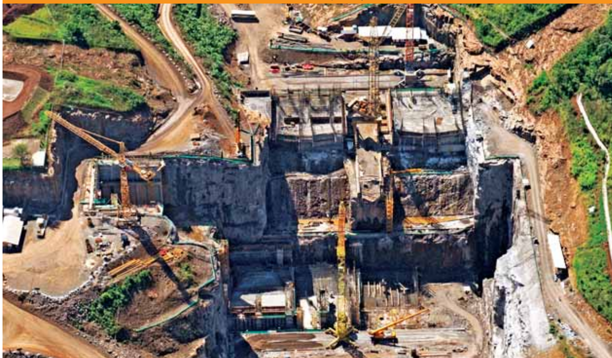
HPP Foz do Chapecó | Construction Power House and Water Intake
