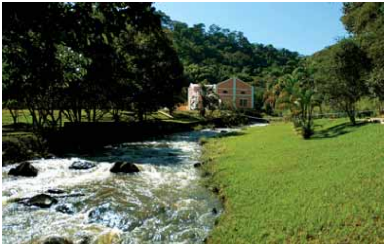
General View of PCH Chibarro | 2.6 MW | São Paulo state
