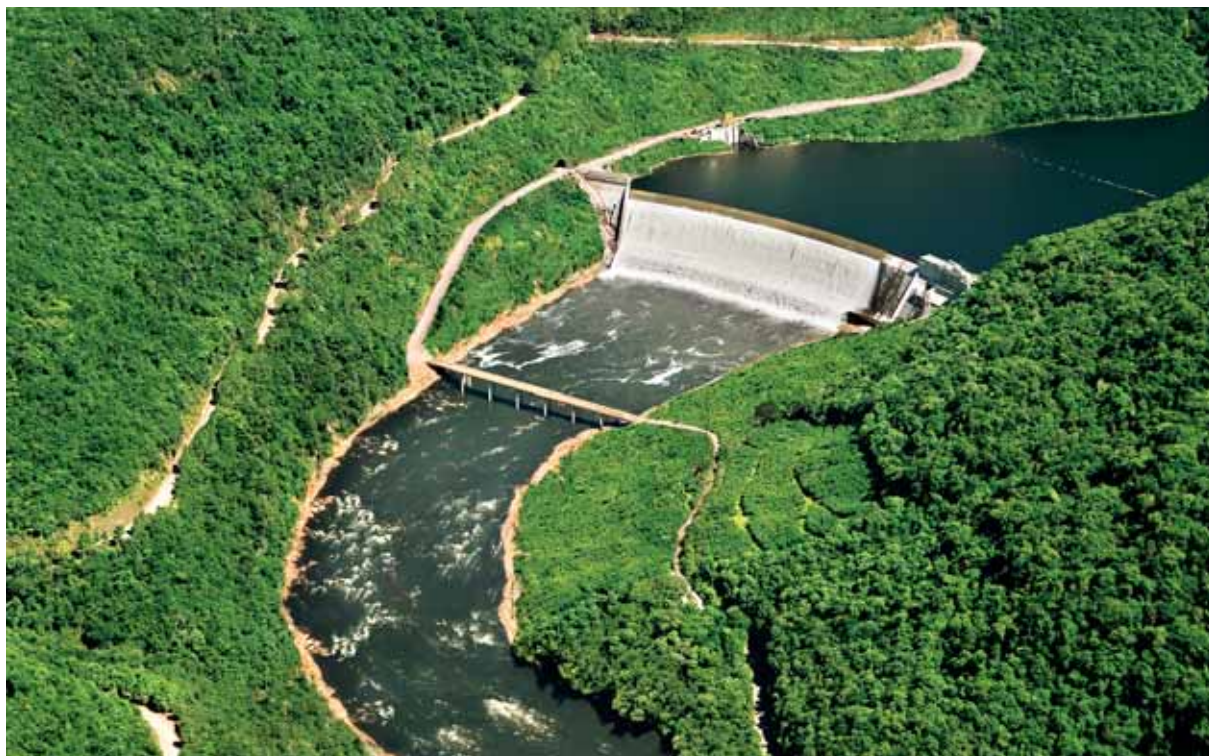
General View of HPP Castro Alves | 130 MW | Rio Grande do Sul state
