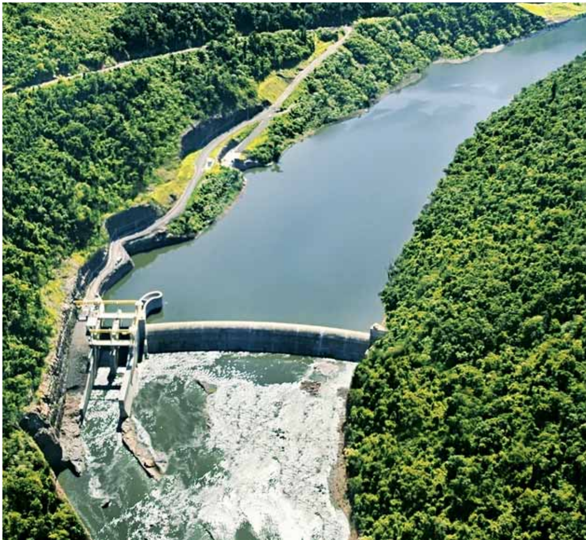
General View of HPP Monte Claro | 130 MW | Rio Grande do Sul state
