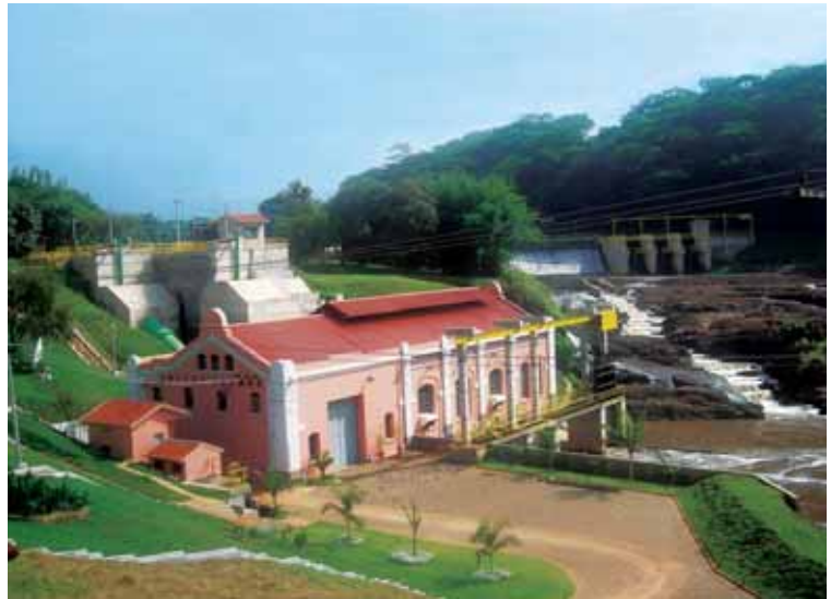
General View of PCH Gavião Peixoto | 4.8 MW | São Paulo state
