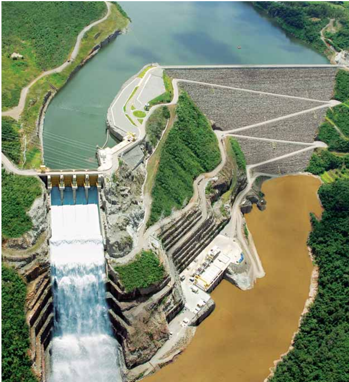
General View of HPP Campos Novos | 880 MW | Santa Catarina state
