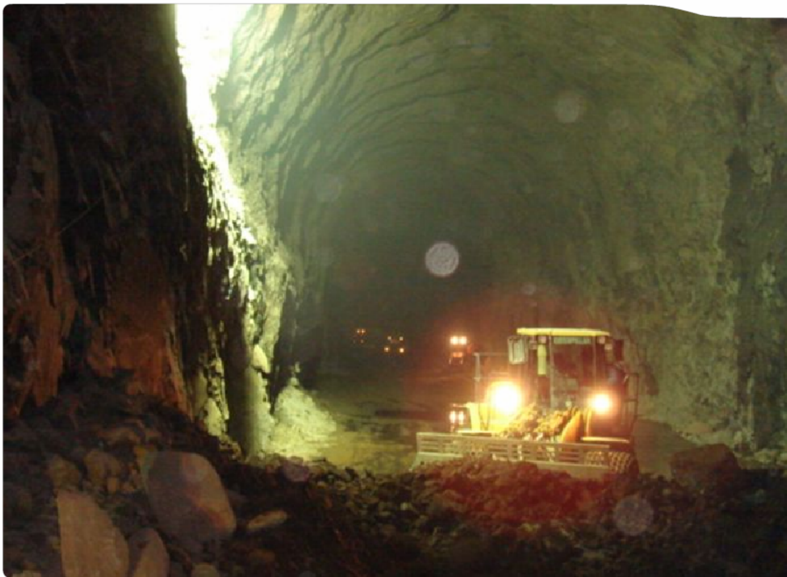
Internal view of the DT1 - removal of the final blocking concrete
