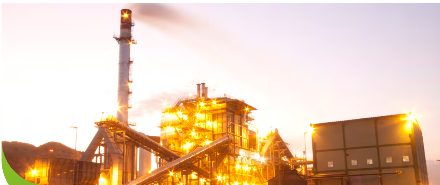
CPFL Renováveis biomass plant in Pirassununga - SP
