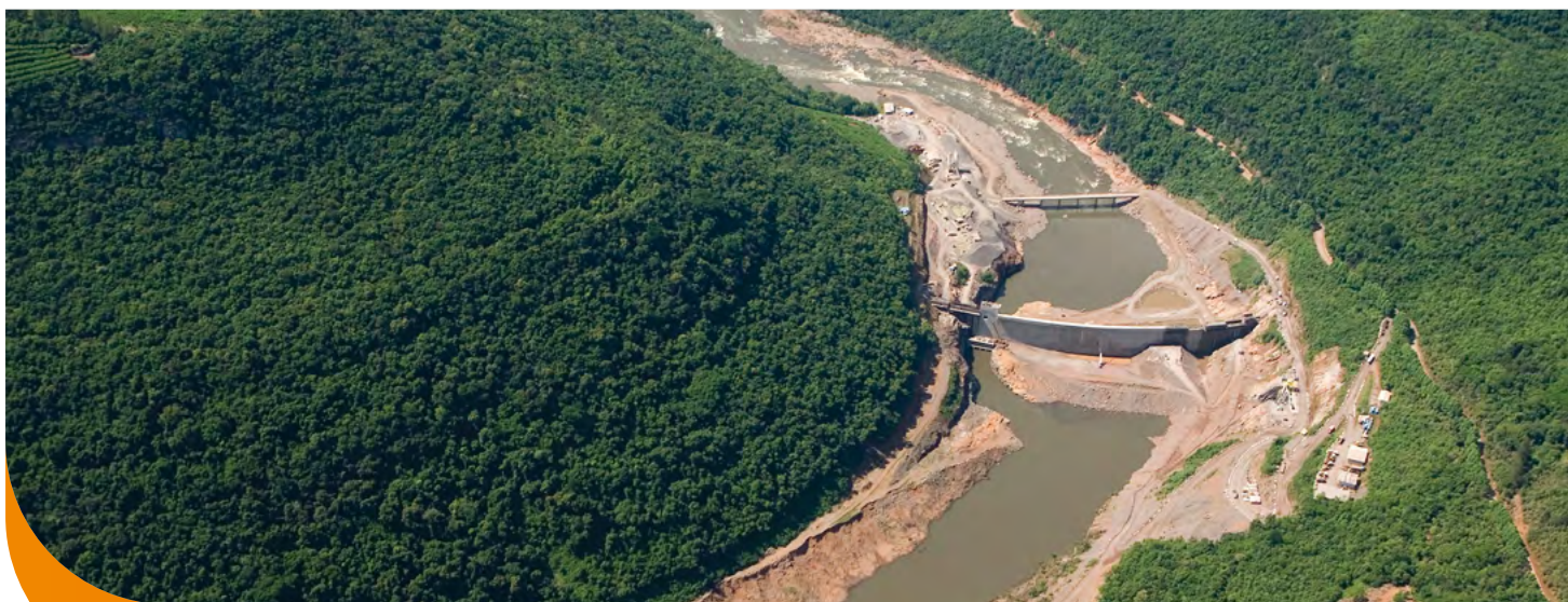
Castro Alves Hydroelectric Power Plant (Ceran)
