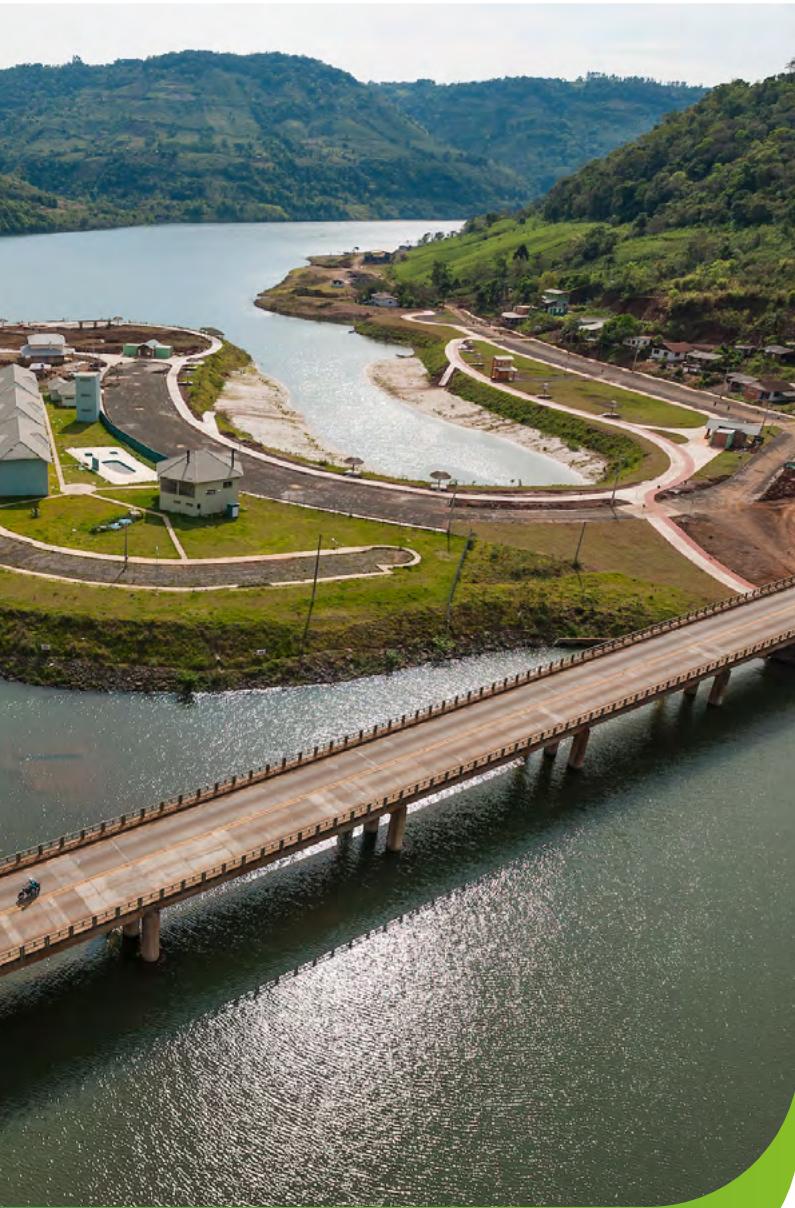
Foz de Chapecó Hydroelectric Power Plant
