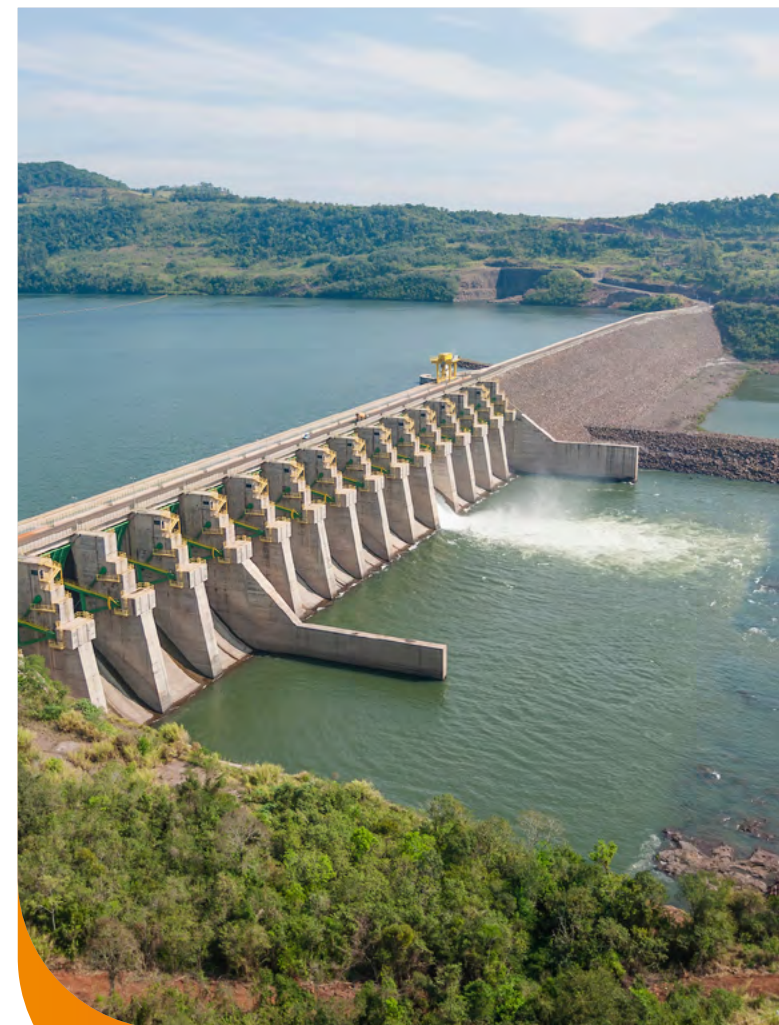
Foz do Chapecó Hydroelectric Power Plant
