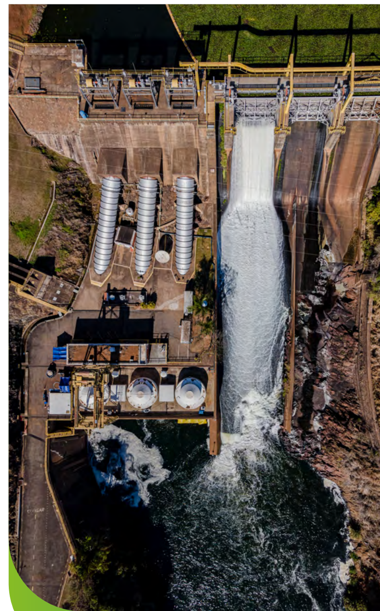
Small Hydroelectric Plant in Americana - SP
