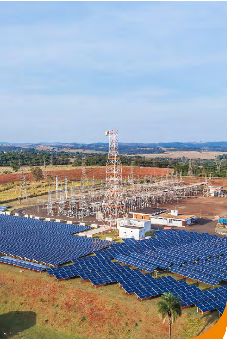
Tanquinho Solar Power Plant - Campinas - SP
