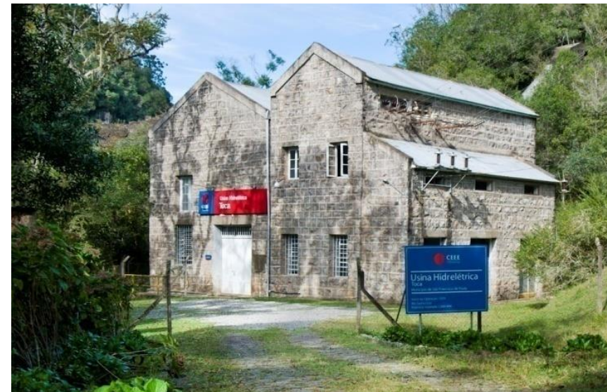
PCH Toca | 1,088 MW | Rio Santa Cruz
