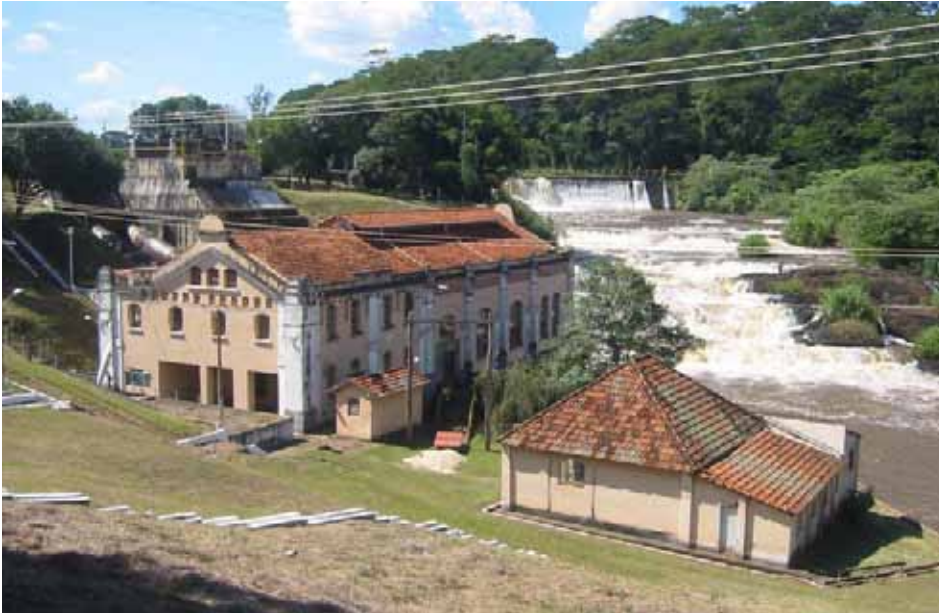
Gavião Peixoto-small hydroelectric power plant | Gavião Peixoto | São Paulo
