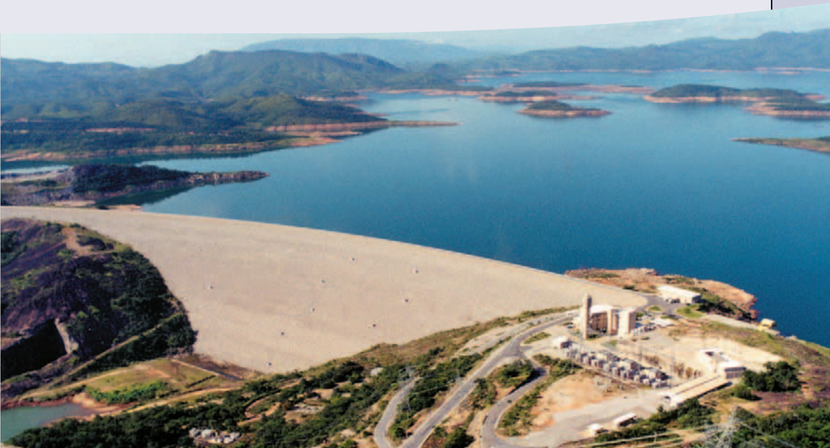
Serra da Mesa hydroelectric power plant | Panoramic view of the Dam and Reservoir | Goiás
