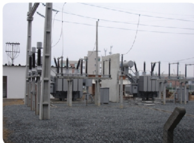
Substation: 138 kV Installed Capacity: 50 MVA
